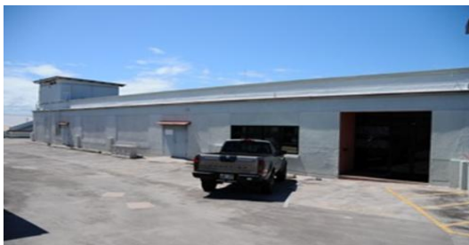
4D parking area & office entrance
